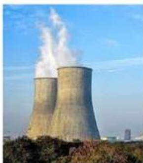
Now on, only about 11% of India's 600 thermal power plant units have to mandatorily install the FGD systems. FILE PHOTO
