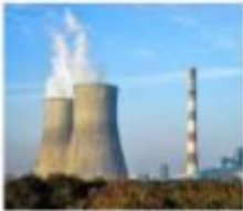
Now on, only about 11% of 600 thermal power plant units in India have to mandatorily install FGD systems. FILE PHOTO
