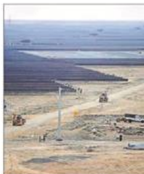
AGEL's operational renewable energy capacity has reached 12,258 MW.
