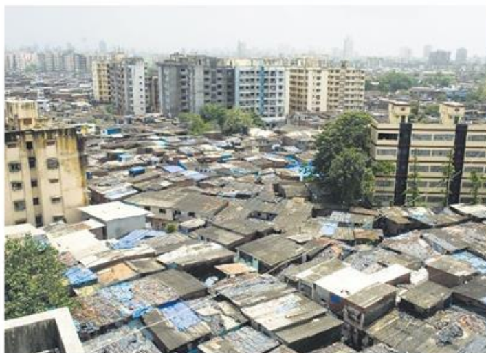
Adani Group said construction was already underway, with significant investments in equipment and manpower for Dharavi's redevelopment. HT
