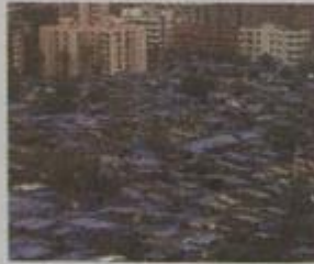
The scheme is going to rehabilitate about 3,700 tenements. File
