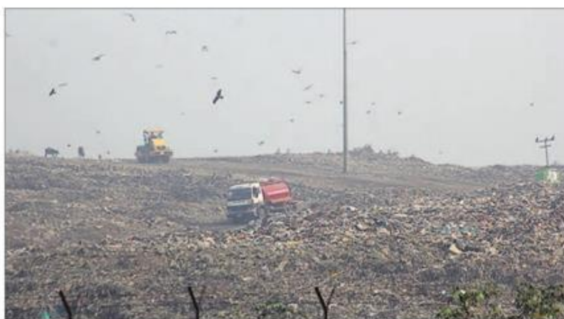
The project involves the bioremediation of 18.5 million tonnes of legacy waste at the landfill. HT PHOTO
